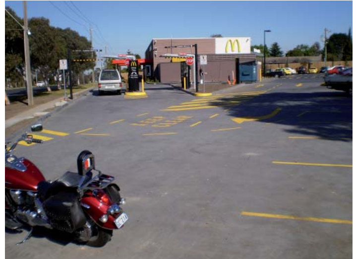
Clayton McDonalds completed carpark Densi-Proof™ for a moisture barrier, body fluid protection, surface hardener and cure & seal.
