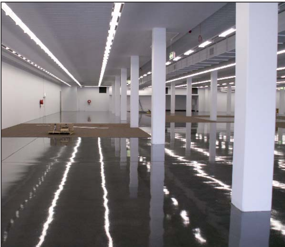
A portion of the interior of a recently completed Spotlight Sydney suburban store showing the Protect Crete, Ardex K15 and Tuffcoat System.
